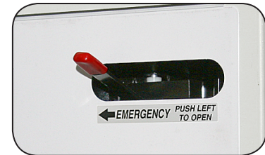
Electric Door Emergency Release
