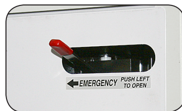
Electric Door Emergency Release
